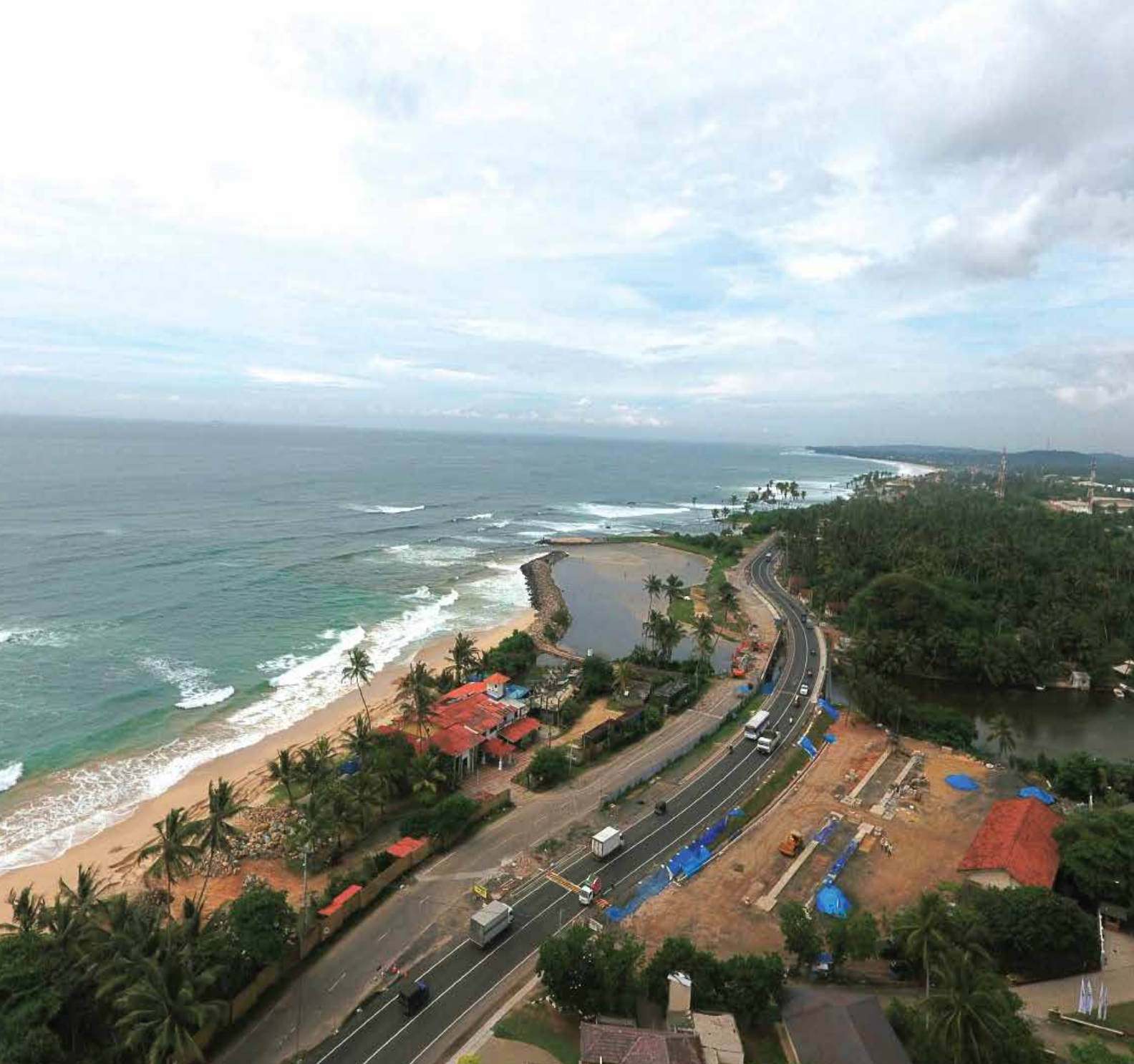
Kathaluwa Bridge construction
