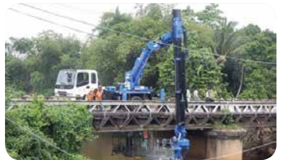
Bridge maintenance vehicle in operation
