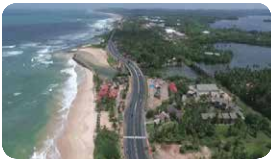
Kathaluwa Bridge nearing its completion
