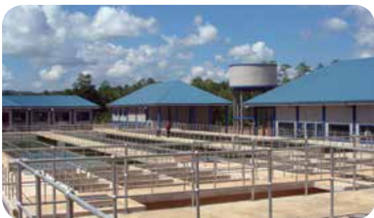
Water treatment facility at Moratuwa
