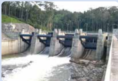
Kukule Ganga Hydroelectric Power Project
