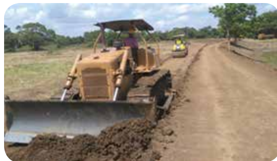
Reservoir bund being rehabilitated as part of the pilot project
